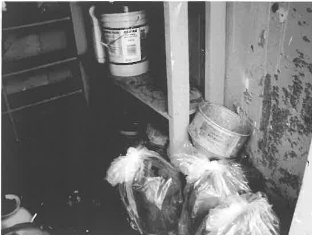
Photo No. 10. Photo of storage containers with flammable liquid located within the flammable storage area.
