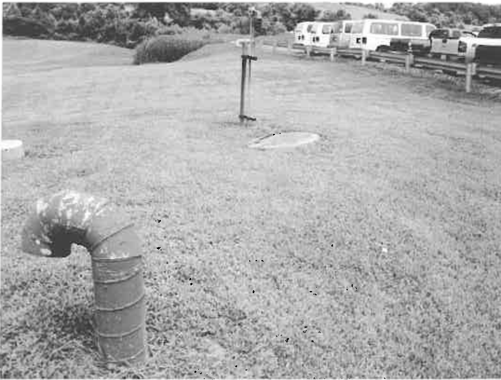
Photo No. 11. Photo of manhole/vault for water service located northeast of UST area.
