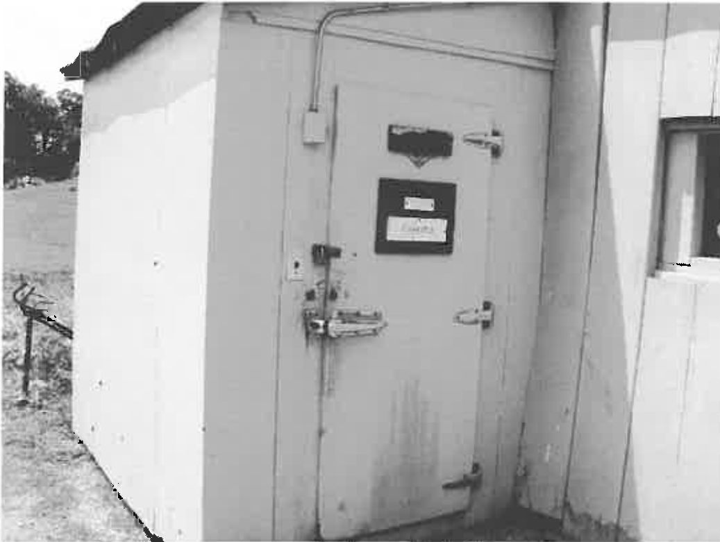
Photo No. 9. Photo of storage area for flammable fluids.
